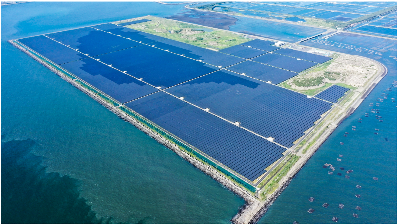
An aerial view of the 272 MW E2 Solar Project in Taiwan
